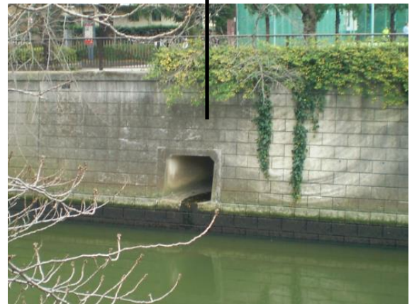
排水渠 (W1.8m × H1.8m)
